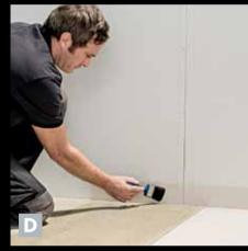
**Stage 2 Waterproofing** First the entire floor and 75mm up the wall is painted with the primer.
