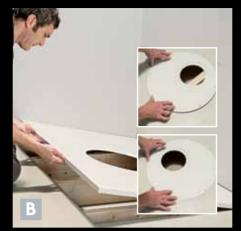
The Aqua-Dec is then placed in the recess to determine where the waste needs to be fitted. Our latest model, the Aqua-Dec EasyFit, has unique drain features\* that allows it to be rotated to avoid any joists that could obstruct the waste. \* Patent No. GB2431341
