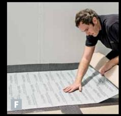
Jointing Tape is also laid in parallel strips to fit below the joins in the Impey membrane, which is then rolled out to cover the Aqua-Dec and the entire floor.
