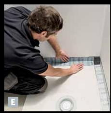
Then all the edges are sealed with the Impey Jointing Tape.
