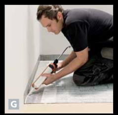
A special additional sealant is then applied to all the corners.
