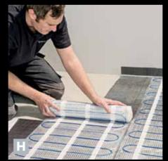
Stage 3 Optional underfloor heating Aqua-Mat<sup>®</sup> underfloor heating comes on a roll of webbed backing that can be laid over the entire floor. This can then be connected to a wall mounted thermostat.
