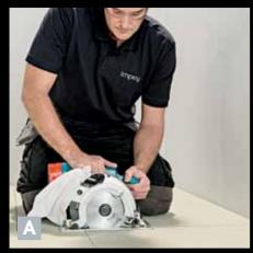
**Stage 1 The Aqua-Dec floor former** After marking the position of the Aqua-Dec floor former, you then cut and remove the floor boards.
